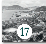
Wanchai looking east
