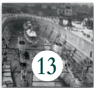
Naval dry dock
